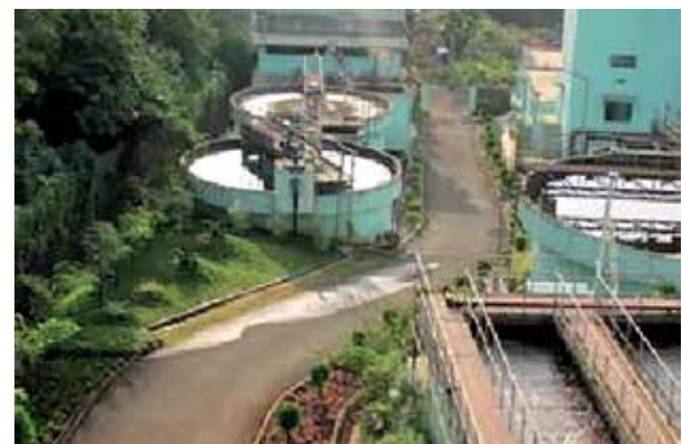
MLD Sewage Treatment Plant
