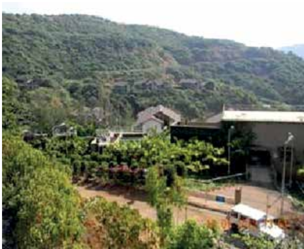
MLD Sewage Treatment Plant
