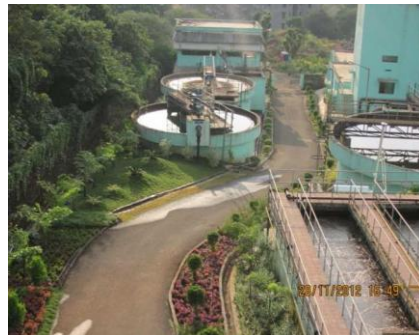
Figure 1 MLD Sewage Treatment Plant
