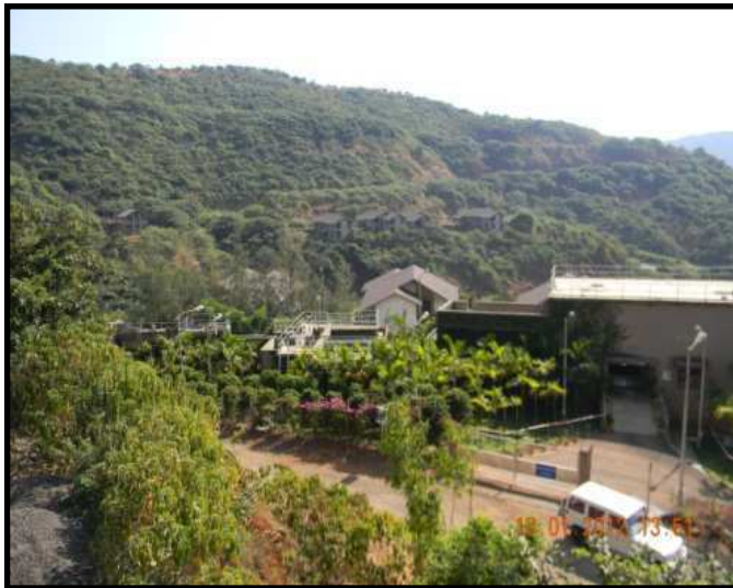
3.4 MLD WATER TREATMENT PLANT
