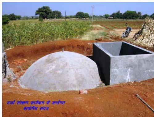
Figure 1 A Biogas Plant under Construction
