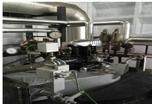
Figure 2: Orai Burner for incorporation of Vegetable Oil Residue
